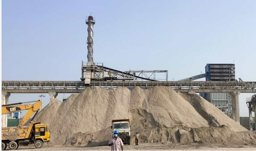
Trucks loading with Excavators
