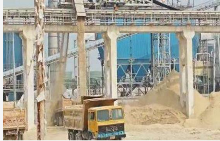
Direct Loading of trucks through feed chutes
