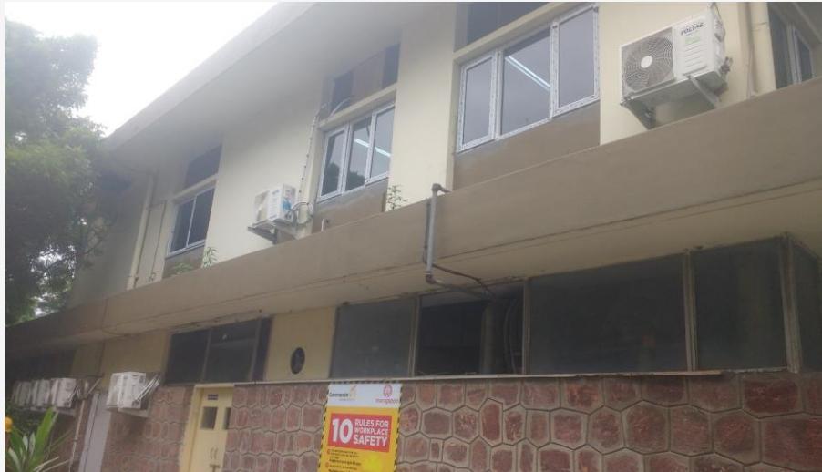
Modernisation of Air conditioners with Energy Efficient 3 Star units
